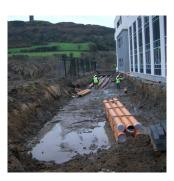
propylene provides excellent heat transfer between the ground and the air. By using the system, it is possible to raise the temperature of air taken in by up to 9K in winter and reduce the temperature by up to 14K in summer.
