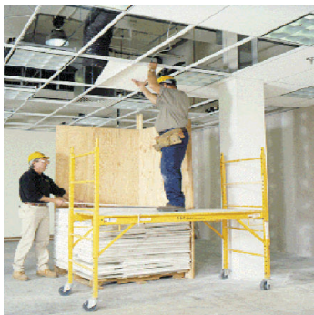
Removal and stacking
