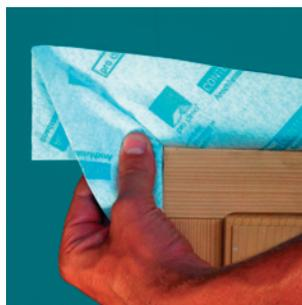
The beginning and end of the pro clima CONTEGA FC is glued with pro clima DUPLEX or ORCON F. The airtight fleece is later embedded in the middle layer of plaster.
