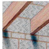
In addition to these benefits, Thermalite Coursing Bricks can also be used for making up between joists.
