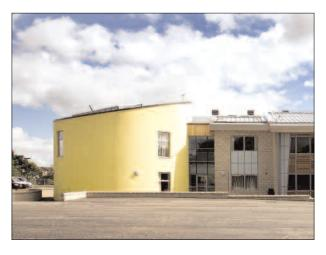
to be self-supporting up to 5m high, enabling them to be used for both the single and two storey wall sections. Using 200mm deep wall panels, Deanburn Primary School was able to achieve an impressive U value for the building walls of 0.15 W/m²K.
