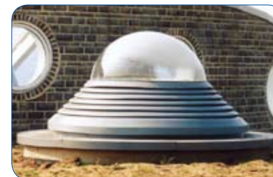
Natures World, Middlesbrough where a 1500mm dia SunPipe system is installed
