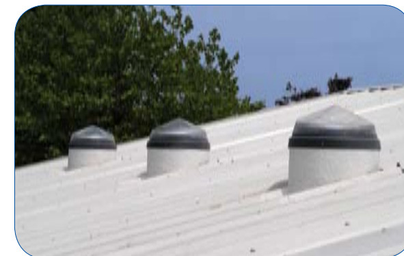
SunPipe flashing detail to metal profiled roof
