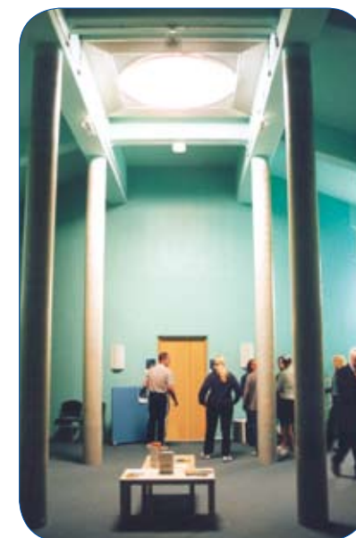
Natures World, Middlesbrough where a 1500mm dia SunPipe system is installed
