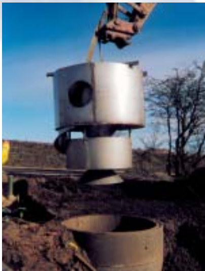
The internal components of the Downstream Defender® manufactured in Grade 304 stainless steel being lowered into the concrete chamber.
