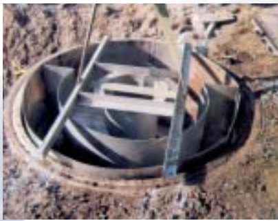
A 1.8m Downstream Defender® being fitted into a standard manhole treating flows from highway runoff.
