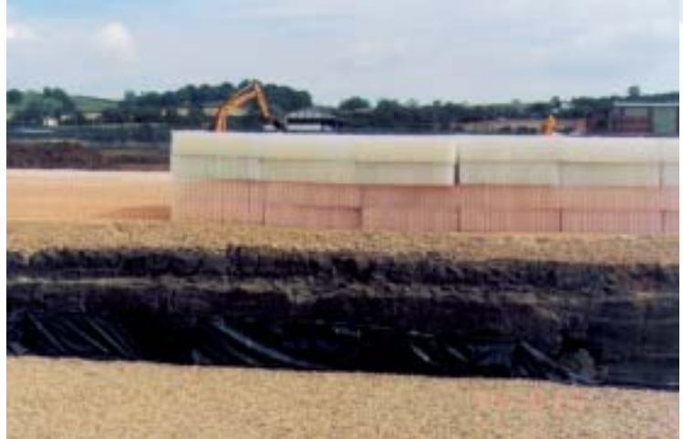
Stormcell® awaiting installation as part of a rainwater recycling system on a Garden Centre.
