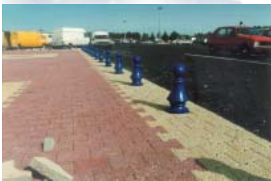
An example of porous paving in France.
