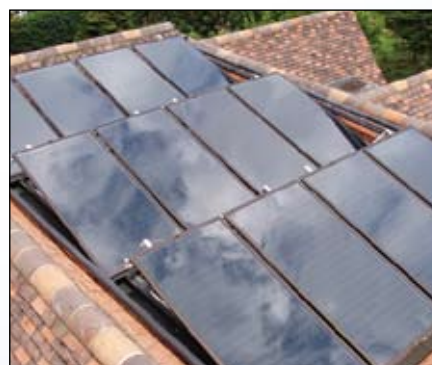
The Burdens Environmental S Class collector - designed as a domestic solar panel capable of being linked up to three in series.
