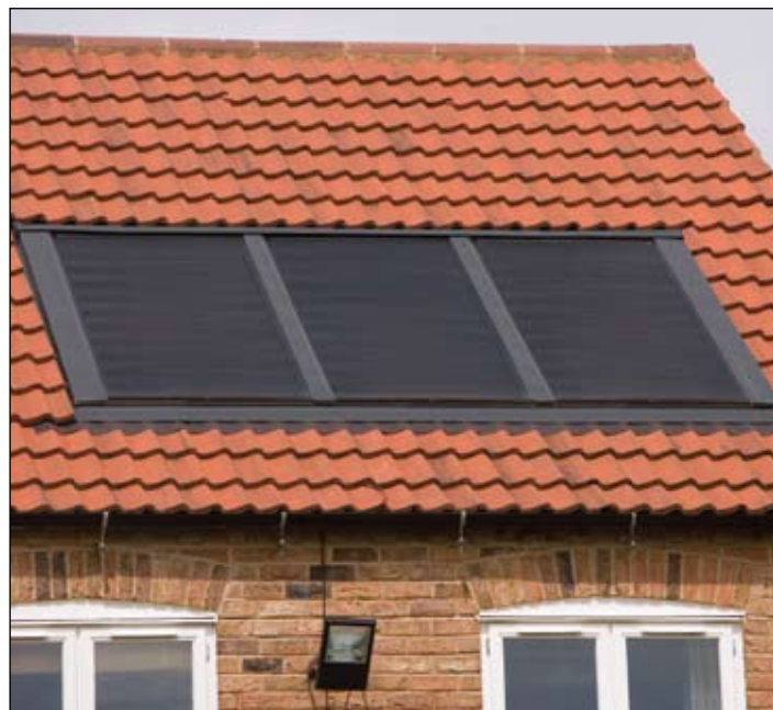
The Burdens Environmental S Class collector - designed as a domestic solar panel capable of being linked up to three in series.
