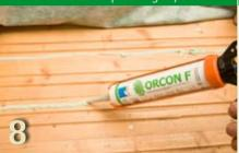
For external rafter insulation with continuous rafters overhanging the eaves, glue the vapour check (e.g. pro clima DA) to two timberboards above the wallplate with two parallel strips of ORCON F. Then stick the two timberboards to the rafters using two parallel strips of ORCON F.
