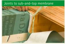
Attach refurbishment vapour check (e.g. pro clima DASATOP) to rough or stone surfaces with a continuous bead approx. 5 mm thick (or more if necessary), incorporating an expansion joint if possible. Do not press the adhesive completely flat. Press the membrane carefully into the corners.
