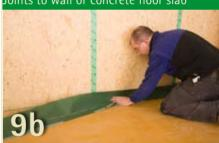
Next, apply a strip of pro clima DA-S and press into the bed of adhesive. Do not press completely flat to allow for structural movement.
