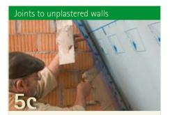
Bed CONTEGA PV in the center of the plaster by pushing back the fleece and reinforcement, applying plaster to the wall behind CONTEGA PV, laying the fleece and reinforcement in the freshly applied layer of plaster and then completing the plaster work – all done!
