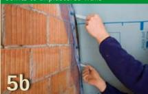
Position the vapour check, then remove the release paper from the back of the CONTEGA PV and affix the fleece to the airtightness layer using the adhesive tape and press to secure firmly.
