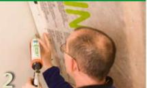
Apply a continuous bead approx. 5 mm thick (or more on rough surfaces). Lay the membrane in place with an expansion joint. Do not press completely flat to allow for structural movement.
