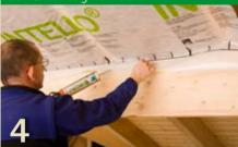
For joints to rough rafters or roof beams, apply a continuous bead of ORCON F approx. 5 mm thick (or more on rough surfaces), incorporating an expansion joint if possible. Do not press the adhesive completely flat.
