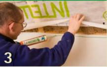
Seal joints in the same way as shown previously for gables. Ensure there is an adequate expansion joint. Do not press the adhesive completely flat.
