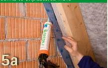
Use CONTEGA PV for well-defined joints to plaster. Attach the fleece as far as possible into the corner using a few dabs of ORCON F, ensuring that there are no voids under the tape.
