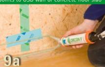
Apply the ORCON F. To save time, apply two beads simultaneously using a double dispensing gun. When crossing RAPID CELL, use a transfer tape such as UNI TAPE or TESCON No.1, as pro clima ORCON F does not stick to RAPID CELL.
