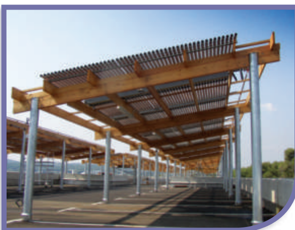
Solar Cooling in Galderma Pharmaceutical Research Centre, France. The 5,600 tubes double up as a car park pergola.
