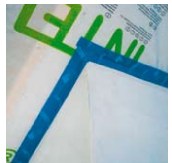
Sticking the vapour check to a smooth, non-porous, non-crumbling, prefabricated chimney using pro clima TESCON PROFIL.
