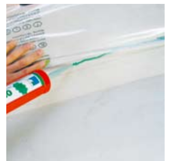
Sticking the vapour check to a cantilever slab using pro clima ORCON F.
