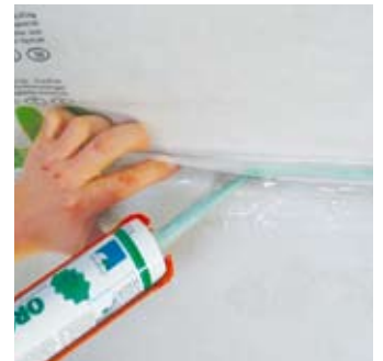
Sticking the vapour check to a rendered chimney using pro clima ORCON F.
