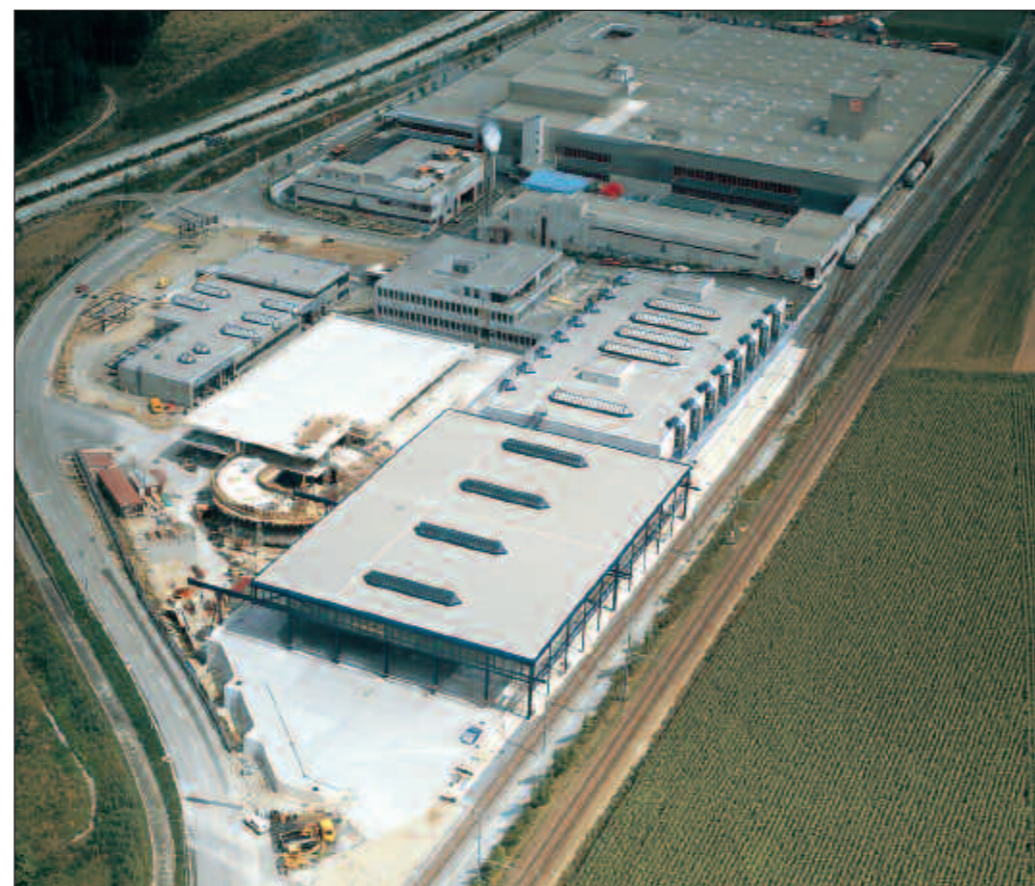
Major Compact Duo-Roof Project.
