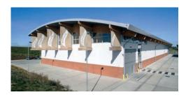
The client decided from the outset that the distribution centre, located in a disused quarry, would be built with a focus on environmental responsibility. This led to the selection of Tradical® hemp lime as the material of choice for the walls of both the 4,400 m² distribution centre and the associated commercial vehicle maintenance facility.
