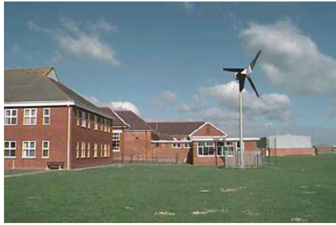
Skegness Gramar School's turbine © Prove Energy
